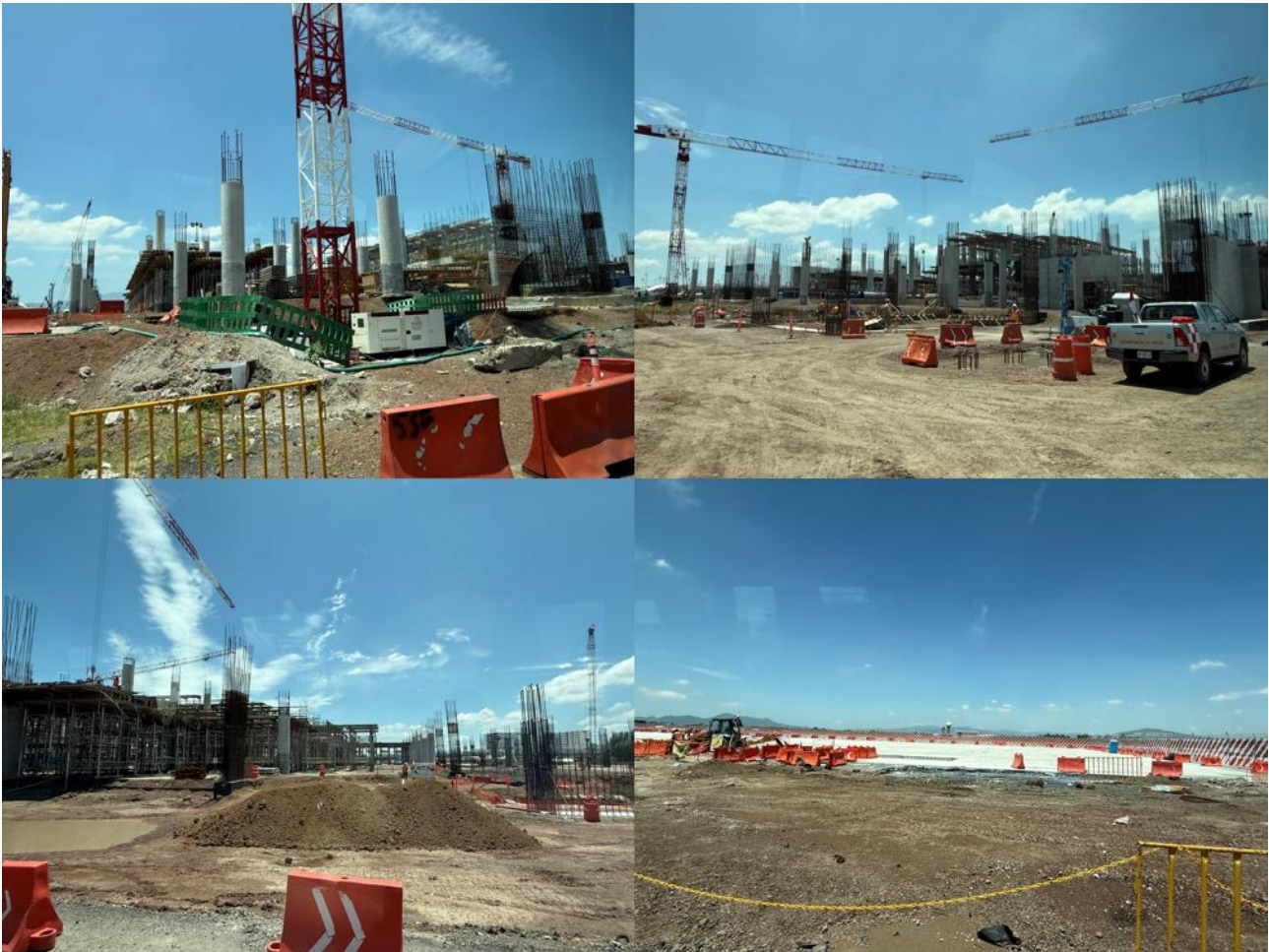
Source – photos from site visit of new Guadalajara Terminal construction
