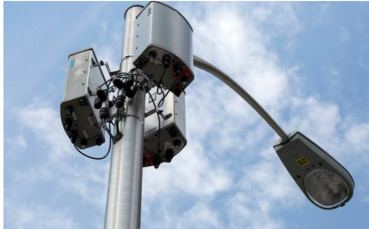
Small cells mounted on street light pole – Baltimore City Council
