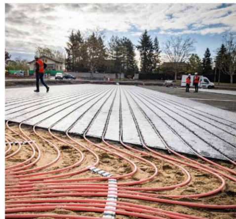
Vinci Eurovia: Power Road
